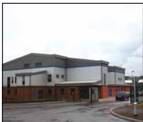
New TA Centre at Pelham Drive, Bootle
