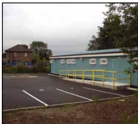
New build project for 1832 (North Manchester) Sqn at Blackley
