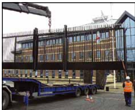
Installation of new electric gates at the RNHQ in Liverpool
